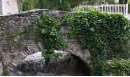
Probably the town’s oldest architectural work of art, dating back to the 11 th century, Sainte-Cécile bridge spans La Foux stream.
